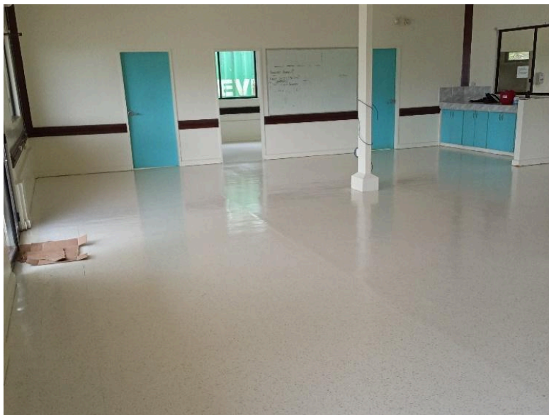
Figure 6. BUILDING J FLOOR RENOVATION, National Campus
