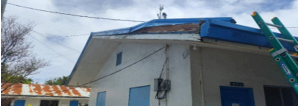
Figure 3. BUILDING I REPAIR, Chuuk Campus
