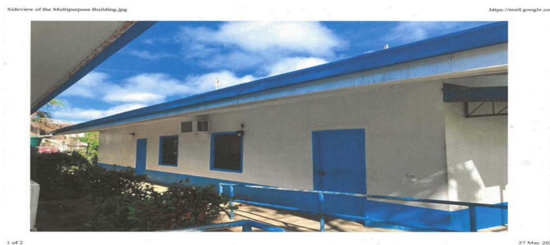
Figure 2. BUILDING H REPAIR, Chuuk Campus
