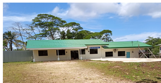
Facilities Improvements – Renovated Building “J” (Former Nursing Center)
