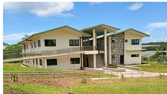
National Campus Student Center (Completed 2026)
