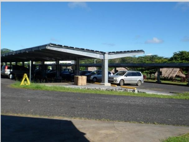
Front main car park with solar panel structure providing dual function of shade and power generation
