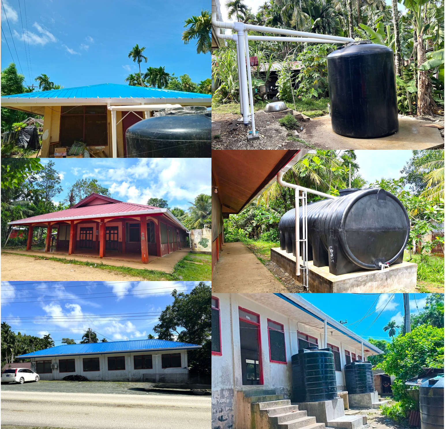
Newly renovated rooftops with integrated rainwater harvesting systems and storage tanks, enhancing water security for three community settlements under the Italian Project
